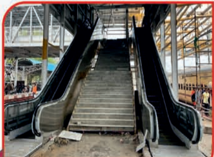
12meter wide Foot Over Bridge at Shalimar Railway Station
