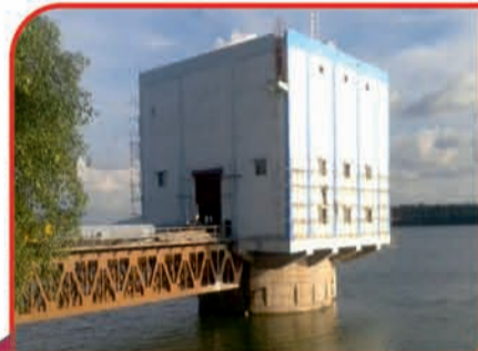
Intake Well At Tilaiya Dam
